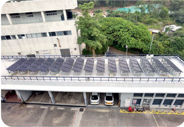
邊界警區總部停車場上方架設光伏板，收集太陽能。 The Border District Headquarters harvest solar energy above its car park using photovoltaic panels.
